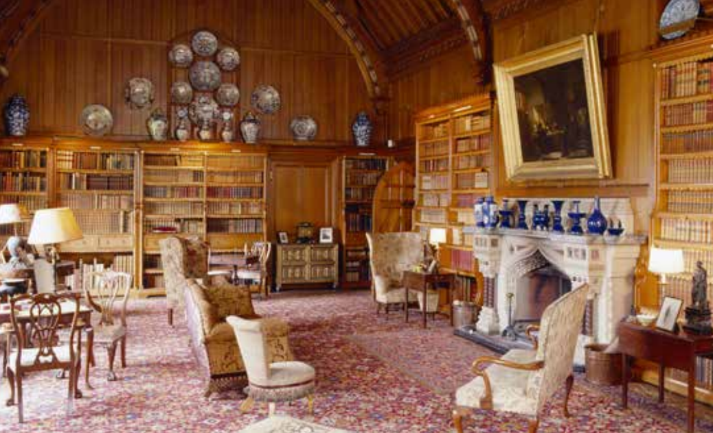
The oak-paneled library with arch-braced collar beam roof.
