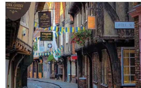
Shambles Rd. in York featuring preserved medieval timber-framed buildings, with jettied floors that overhang the street.
